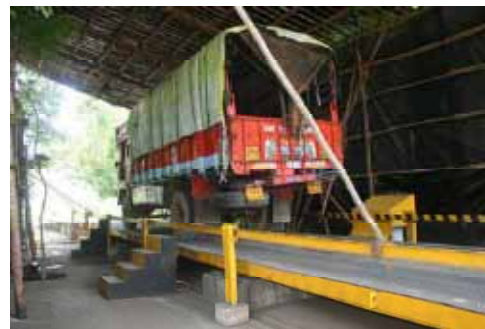
The 100-ton weighbridge built on a stilt to protect load cells during monsoon
